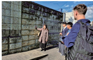
wall of the Church made by Oya-ishi
