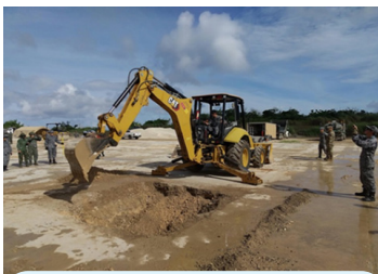
The explosion site is being restored by JASDF
